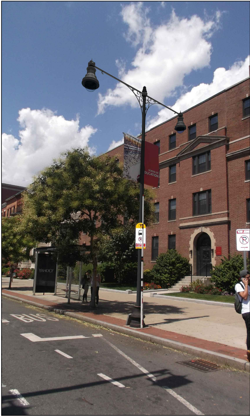
EXISTING PHOTOGRAPHIC VIEW
