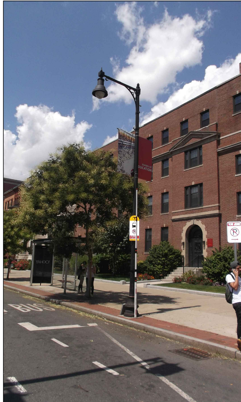
EXISTING PHOTOGRAPHIC VIEW
