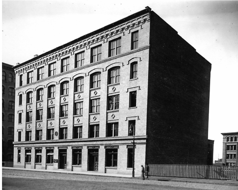
Fig. 4. Example of tripartite façade, with a base, arcaded midsection, and “capital” top floor accentuated with a brick dentil cornice. Photo of 312-320 Summer Street, c. 1905.
