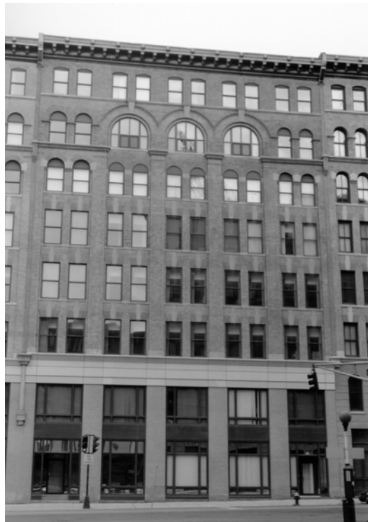
Fig. 7. Summer Street wool warehouse in high-style Classical, 256-260 Summer Street.
