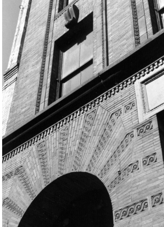
Fig. 5. Classical Revival in the high style, detail of 348-352 Congress Street, 1894.
