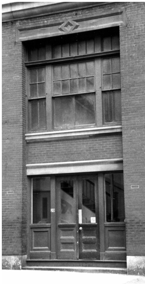
Fig. 23. Detail of original doorway with double-leaf, paneled, wood doors and original window. Photo of 20 Melcher Street.
