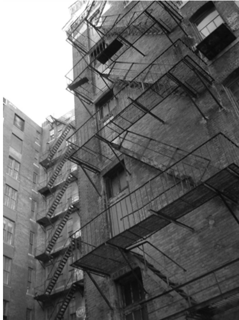
Fig. 22. Typical fire escape balconies and stairs in Fort Point Channel.
