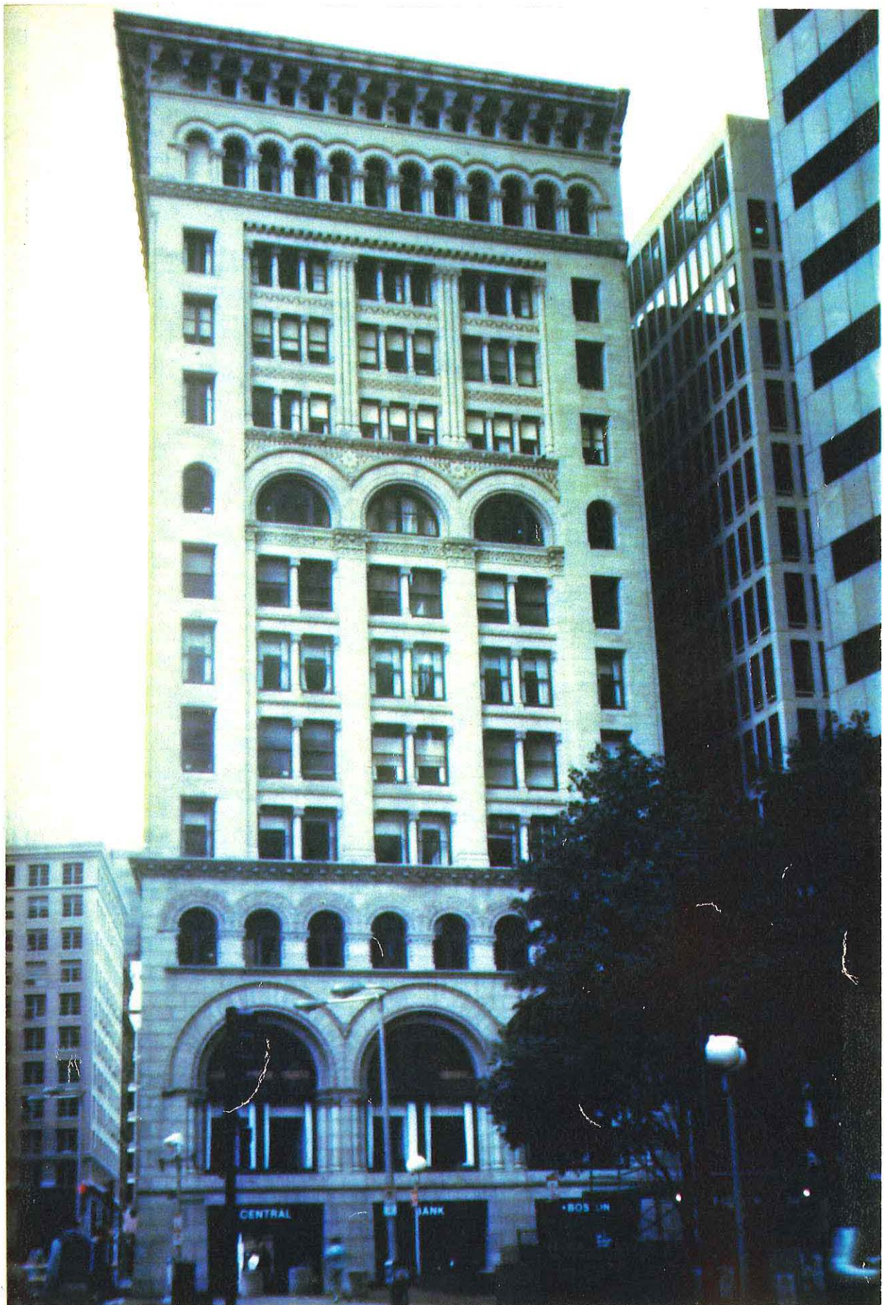
The Ames Building, Washington Mall elevation, c. 1986.
