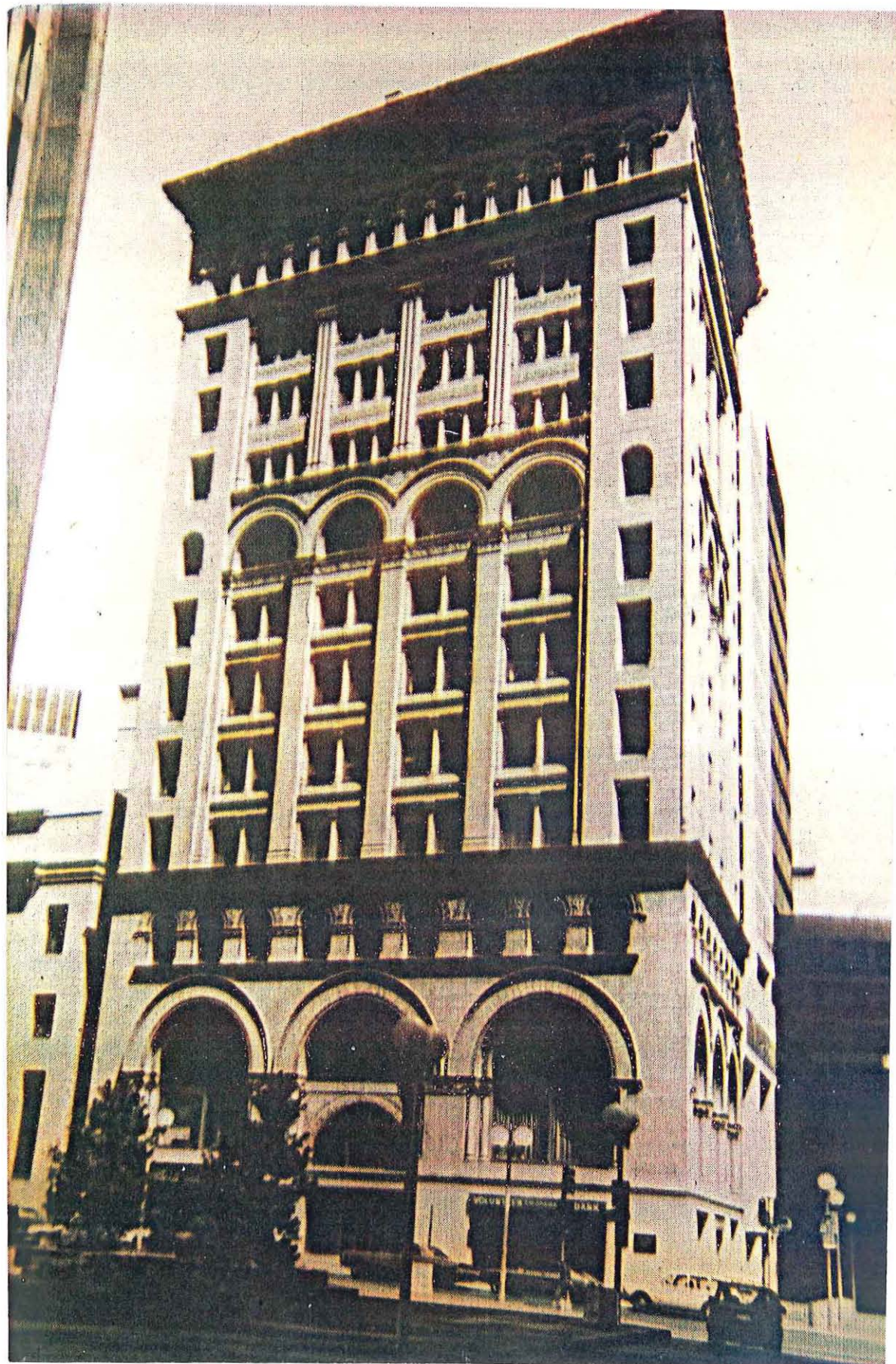
Ames Building, Court Street elevation, c. 1960.
