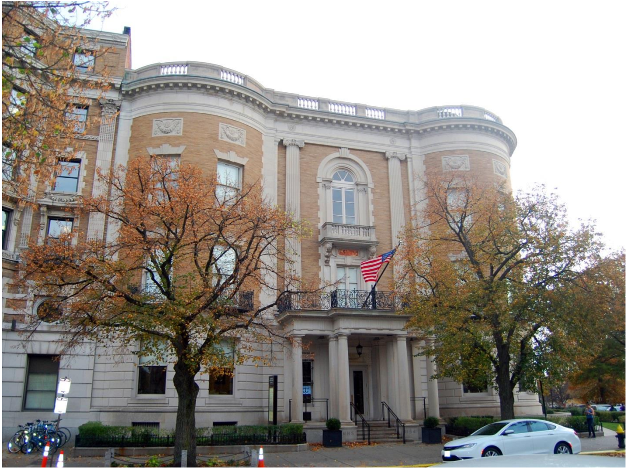
Figure #2. The primary (north) façade of the Massachusetts Historical Society Building on Boylston Street (looking south), November 2015.
