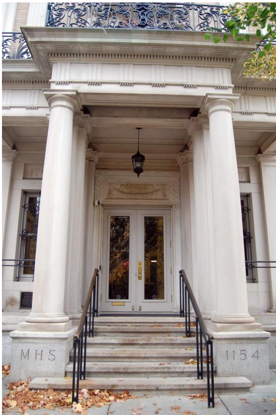
Figure #4. View of the portico on the Boylston Street elevation (looking south), November 2015.
