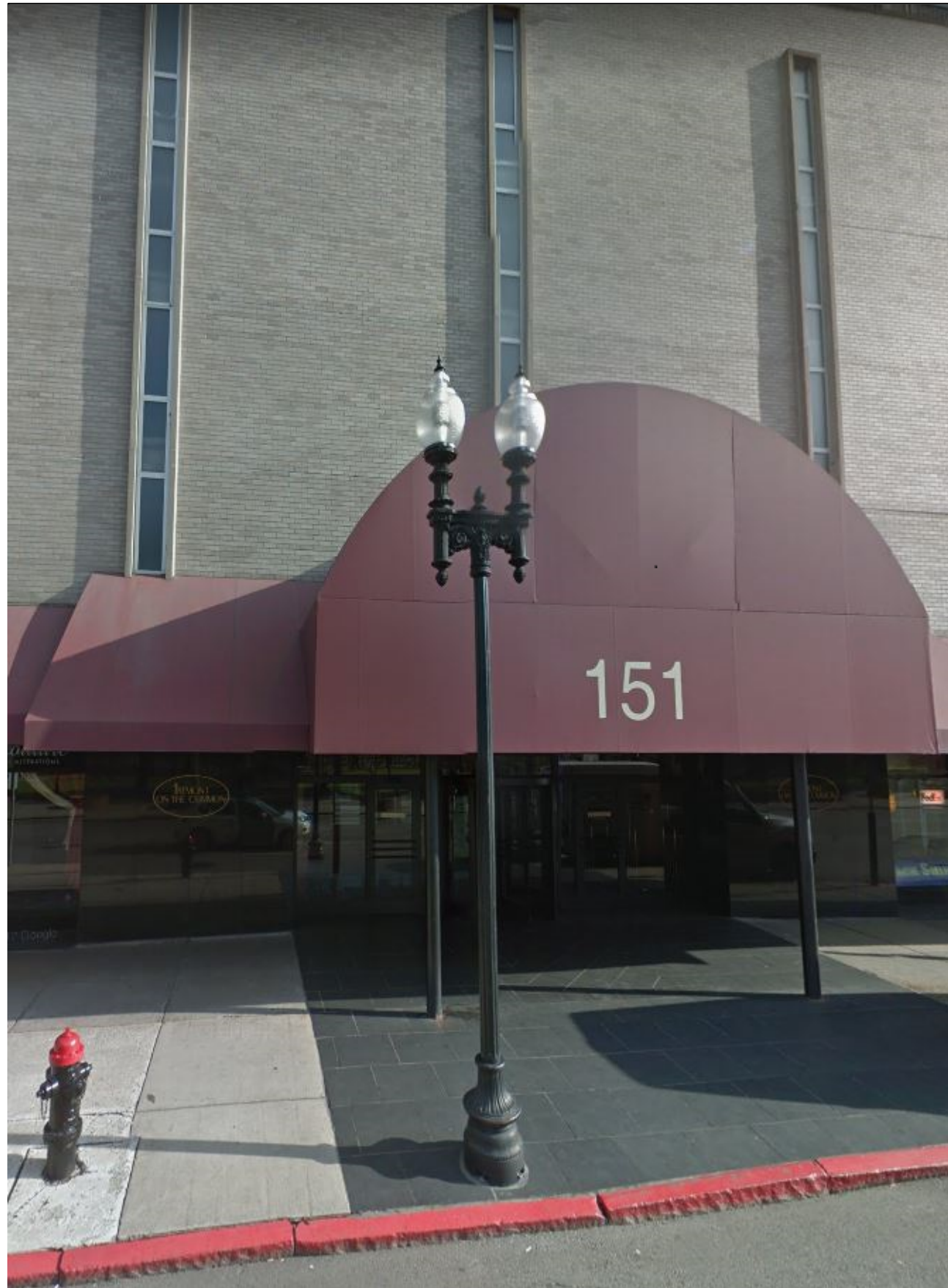
EXISTING PHOTOGRAPHIC VIEW
