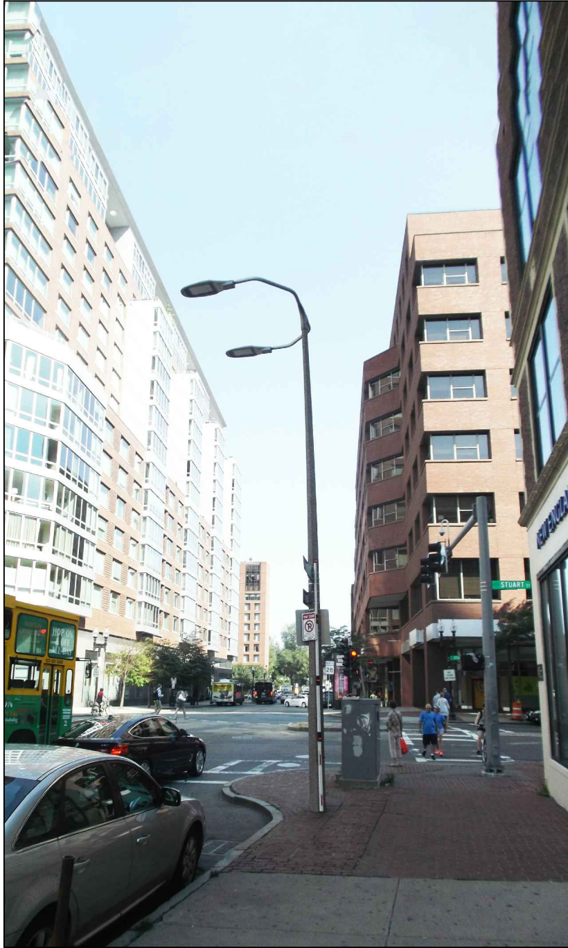
EXISTING PHOTOGRAPHIC VIEW
