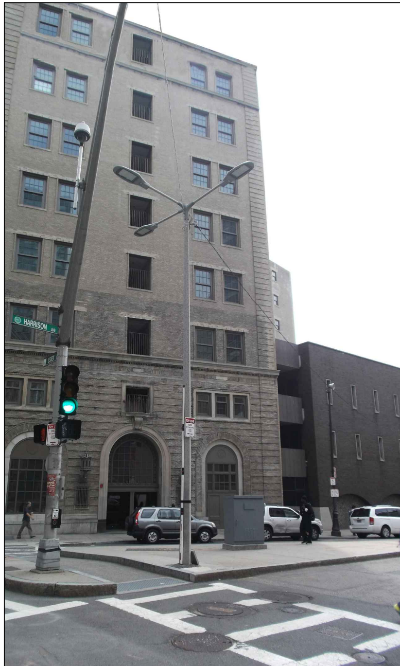
EXISTING PHOTOGRAPHIC VIEW
