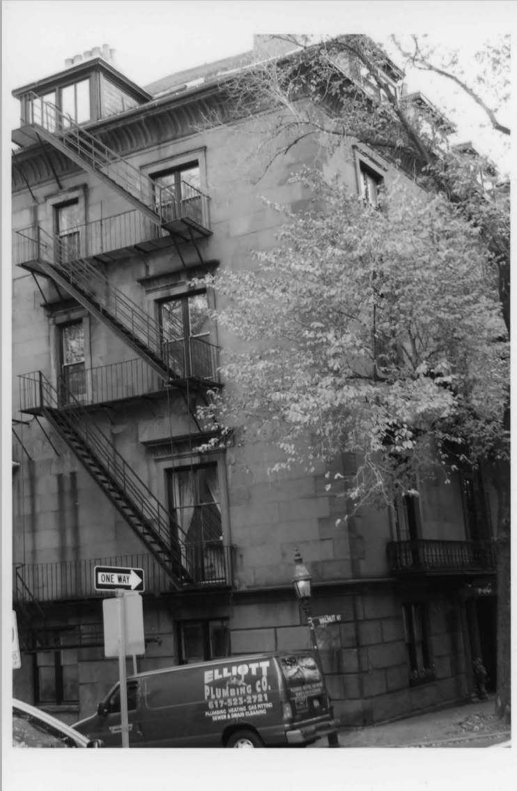
SS 31. 40,42 Mt. Vernon St. Ed Gordon 4/06 Facing SW
