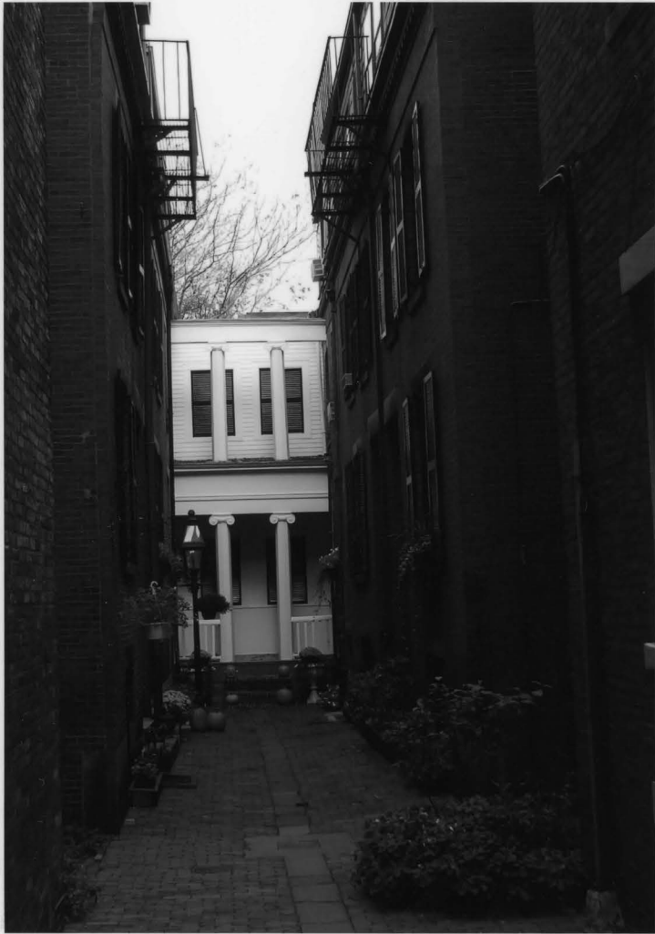
NS 19. 1 to 6 Rollins Place Ed Gordon 11-05 Facing N
