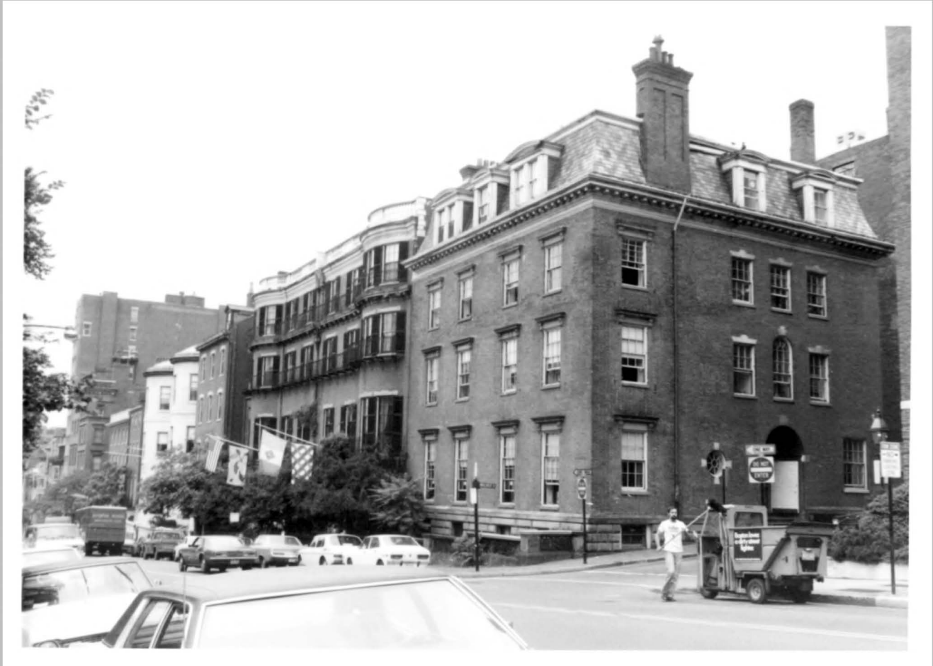
4. Beacon Street looking west from Joy Street.
