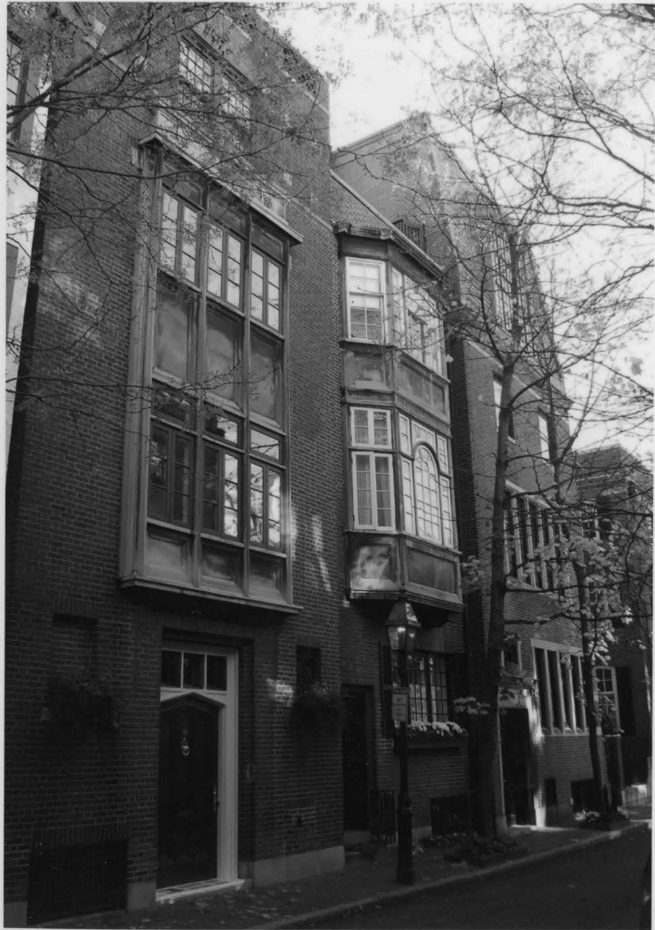
F41. 32, 34, 36 Lime St Holmes 11-05 Facing SW
