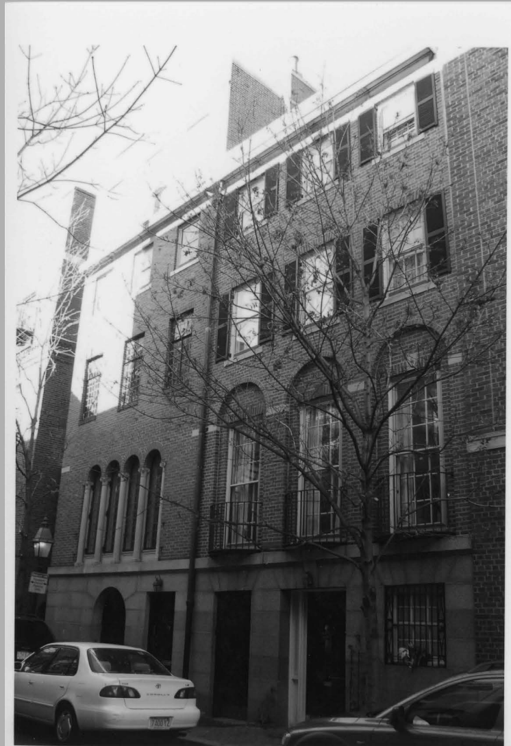
F42. 24, 26, 28, 30 Lime St Holmes 11-05 Facing SW
