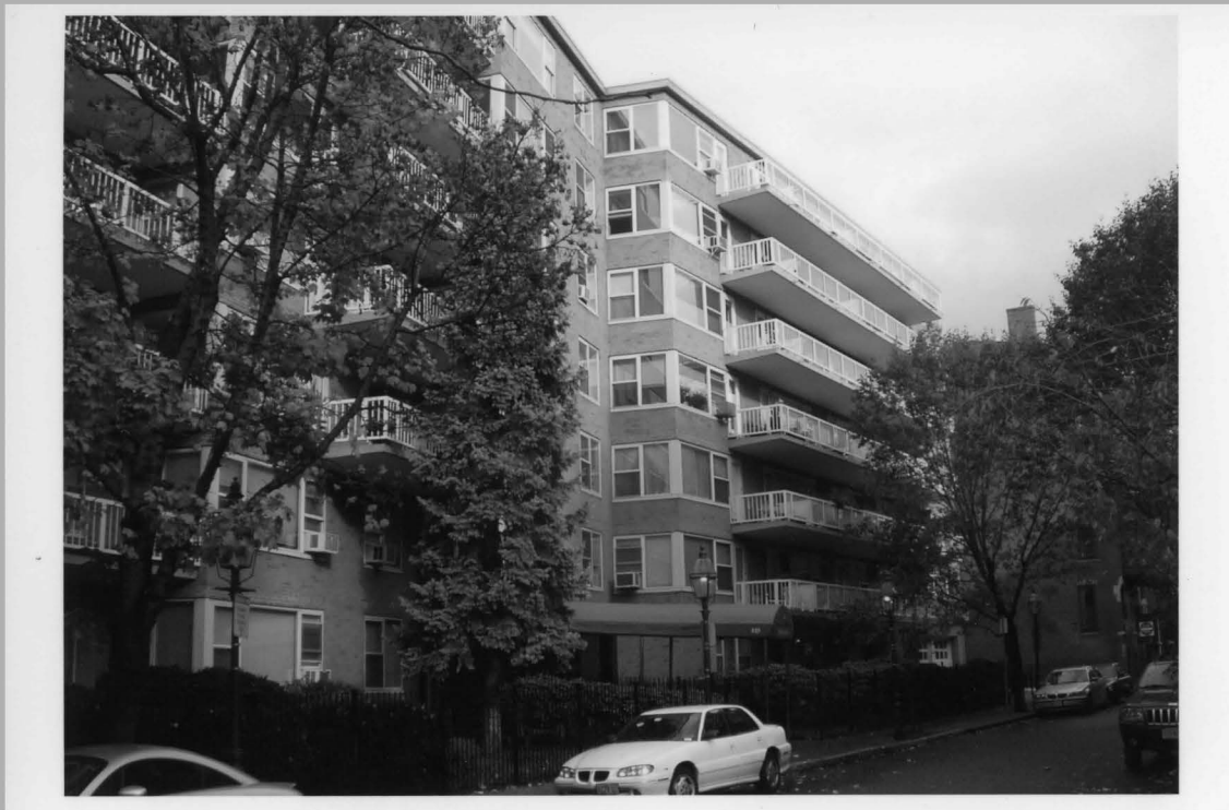
F8. 145 Pinckney St J. McCarthy 11-05 Facing E (River House Apartments)
