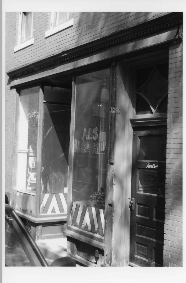
NS 30. 12 Grove St (Detail) Ed Gordon 4-06 Facing NE
