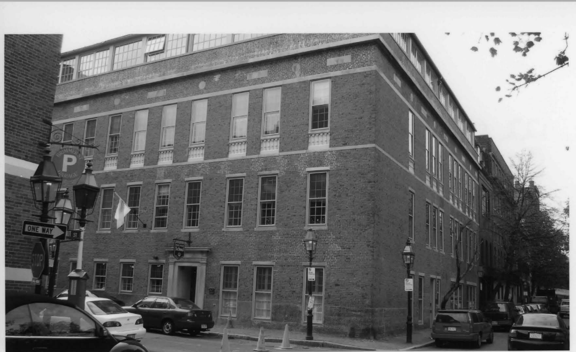
F26. 122 Chestnut St Holmes 11-05 Facing SW (Park Street School Apartments)
