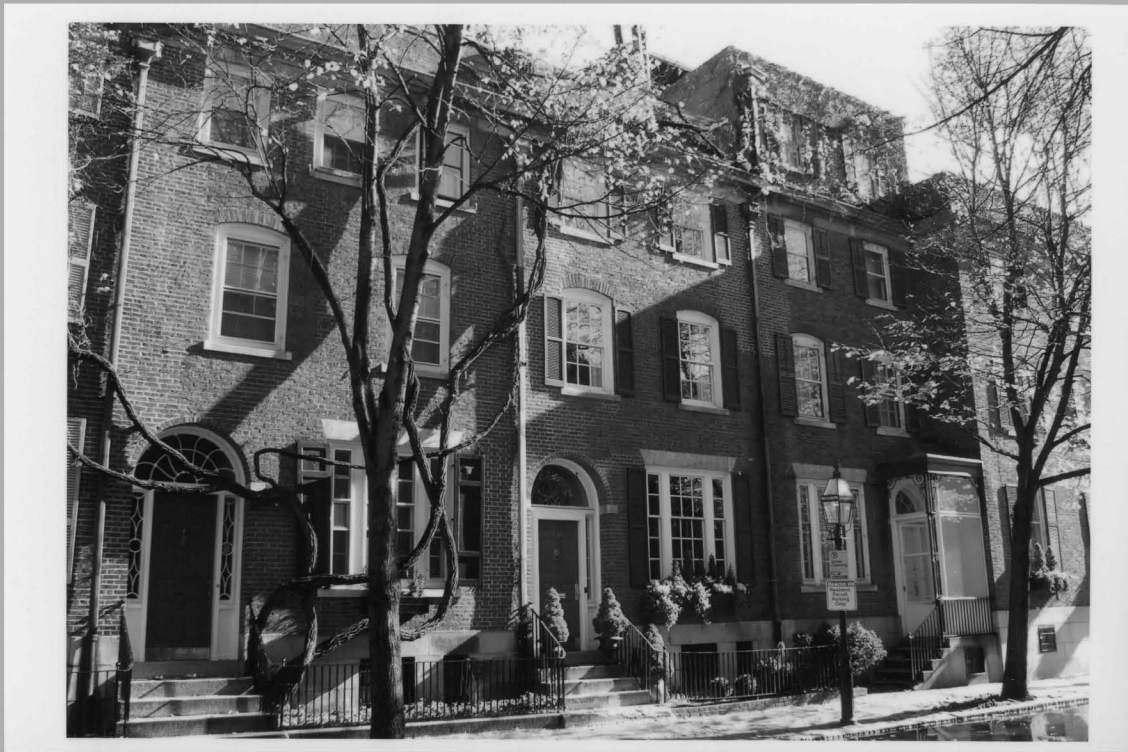
F39. 54, 56, 58 Brimmer St Holmes 11-05 Facing SE
