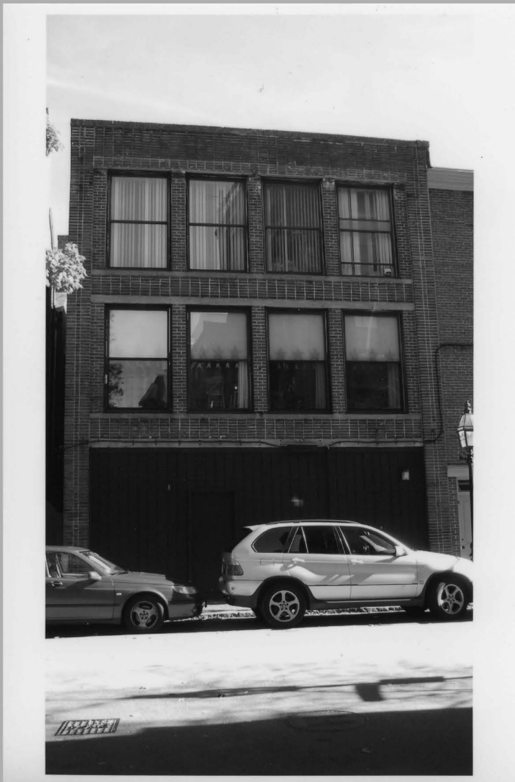
F47. 57 River St Holmes 11-05 Facing E
