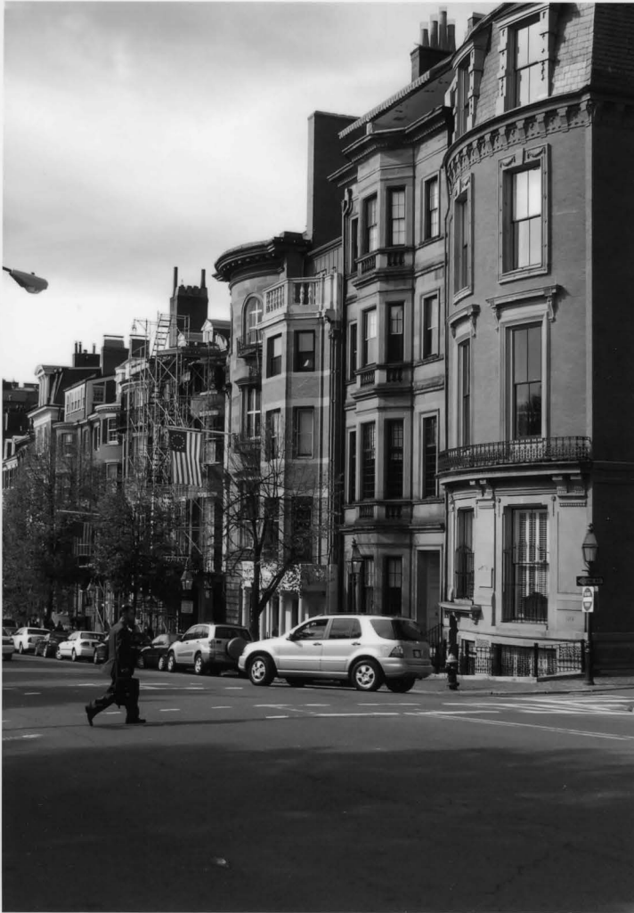
SS 09. 50 to 63 Beacon Street Ed Gordon 10-5 Facing NW
