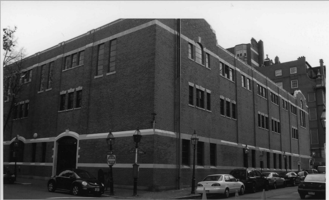
F25. Chestnut & Brimmer Sts Holmes 11-05 Facing SE (Brimmer Street Garage)
