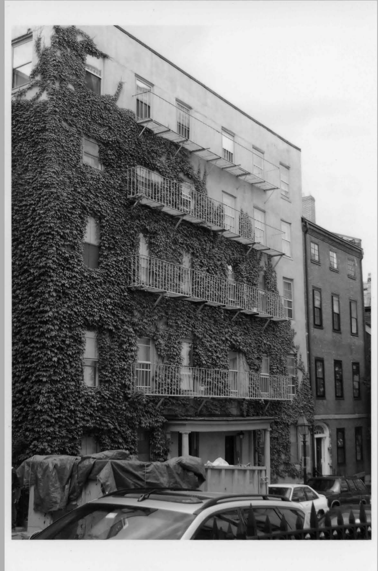
SS 60. 65-67 Hancock St. Ed Gordon 5/06 Facing NW
