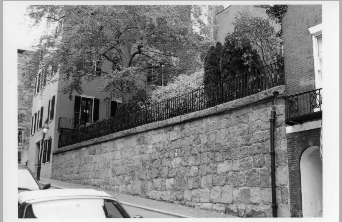
SS 32. 14 Walnut St. Retaining Wall Ed Gordon 4/06 Facing NE
