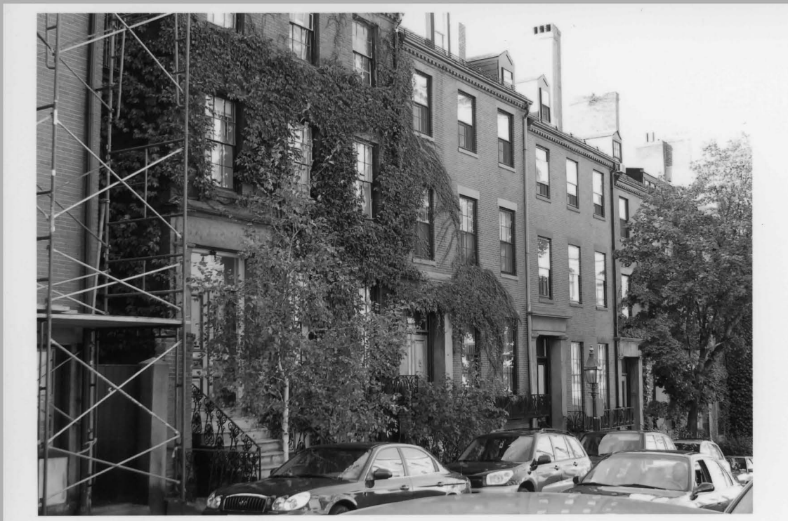
SS 26. 75,77,79 Hancock St. Ed Gordon 10/06 Facing NW
