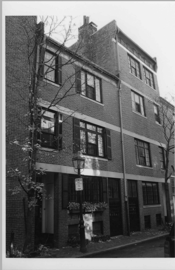
F44. 4 & 10 Lime St Holmes 11-05 Facing SW
